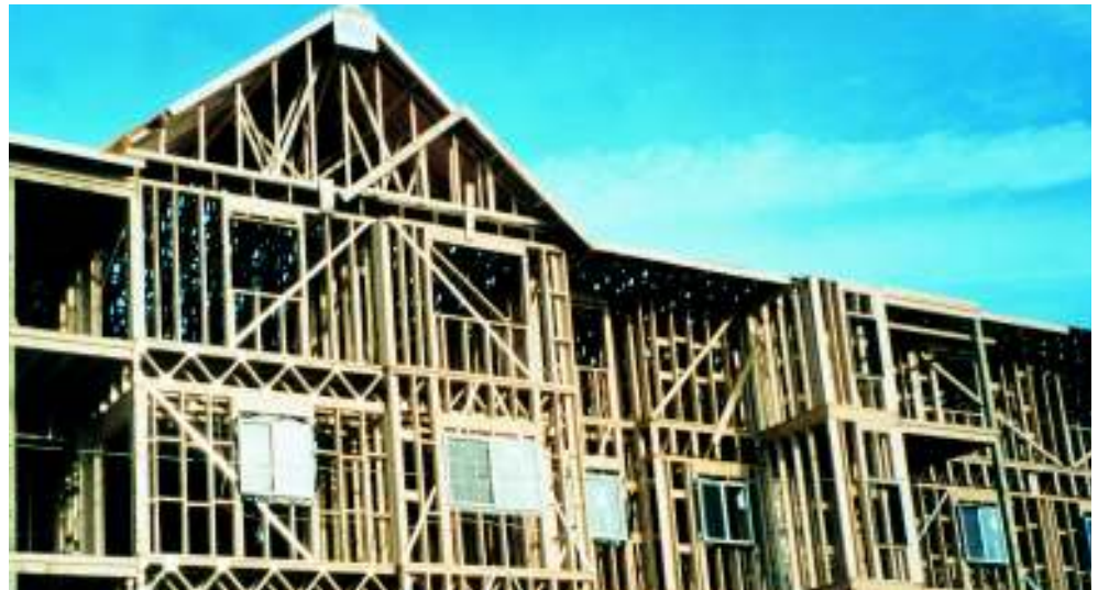
PHOTO 6: Wood-frame construction meets building code requirements for safe housing.
