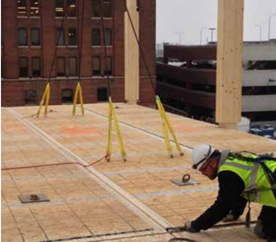
Figure 7.4: Installed roof panels with gaps for expansion. (Photo courtesy of StructureCraft Builders Inc.)
