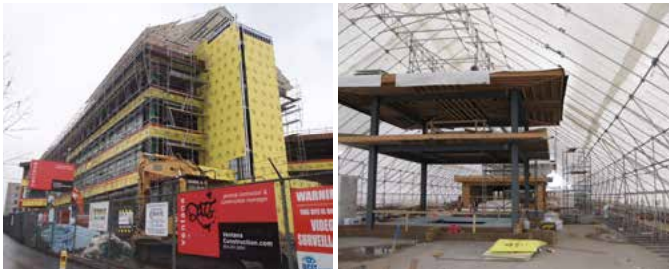
Figure 7.9: Fixed tenting installation. (Photos courtesy of Fast+Epp)
