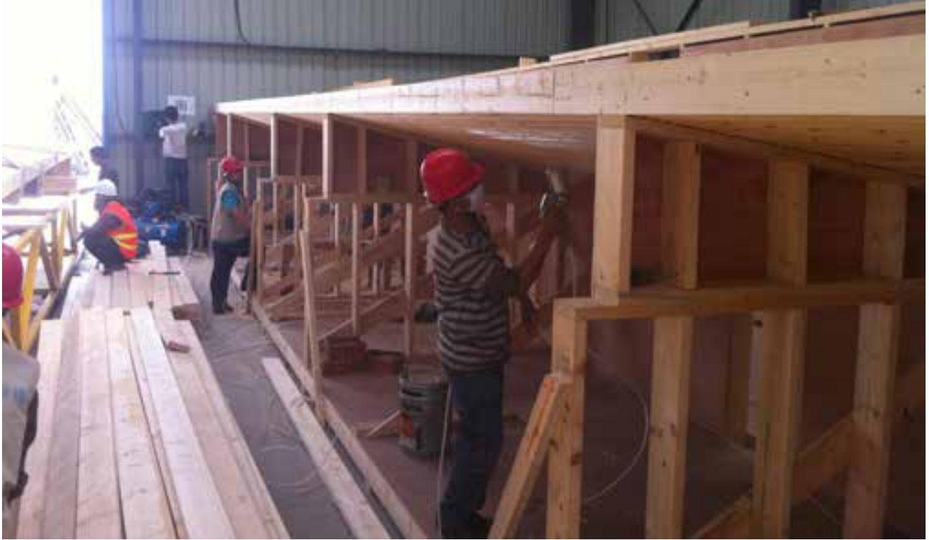
Figure 6.4: Shop applied coating on NLT. (Photo courtesy of StructureCraft Builders Inc.)
