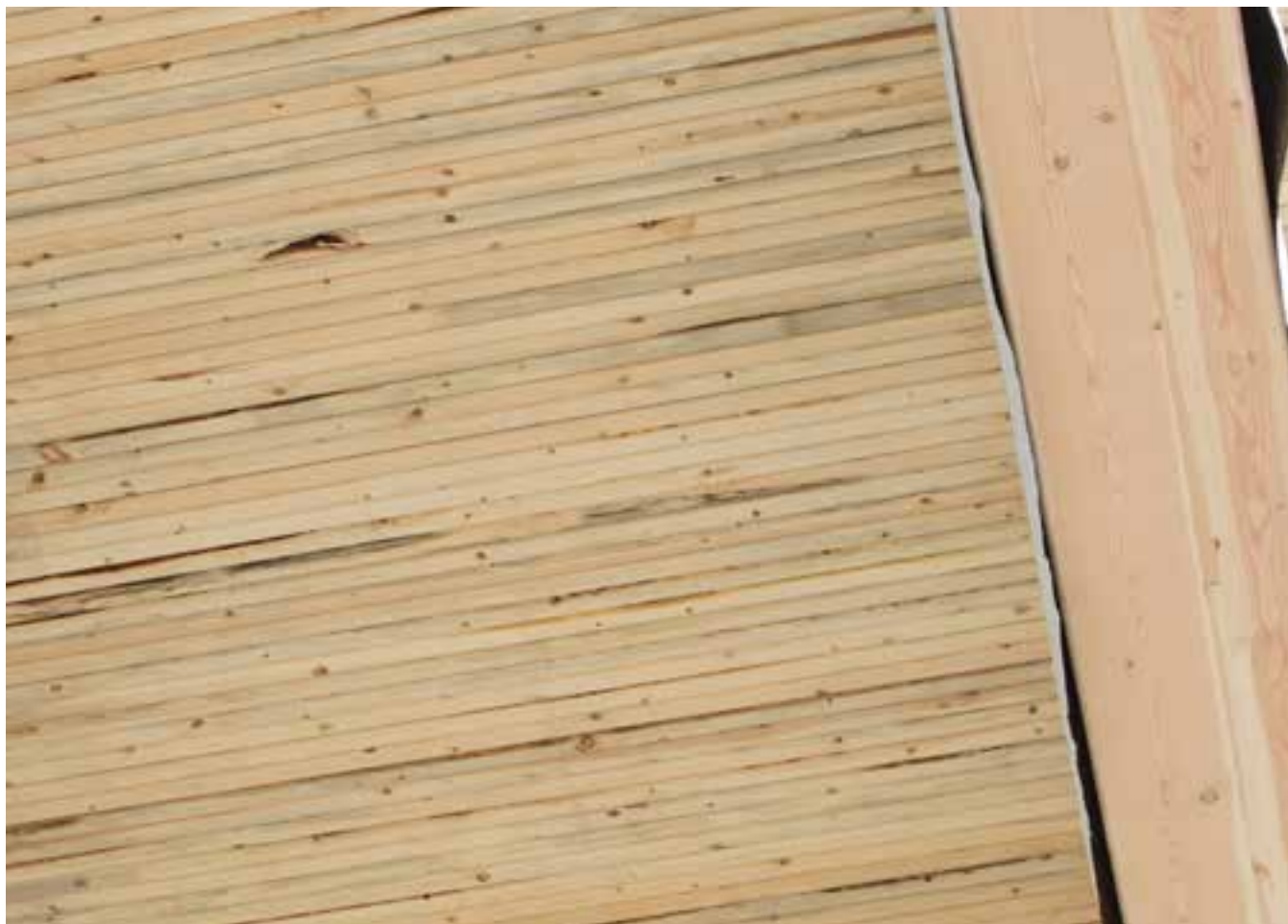
Figure 6.1: NLT showing blue staining from beetle-killed wood. (Photo Courtesy of Perkins+Will)
