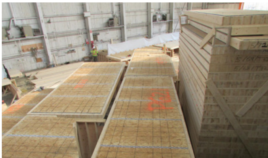
Figure 7.2: Storage set up with dunnage and stickers. (Photo courtesy StructureCraft Builders Inc.)
