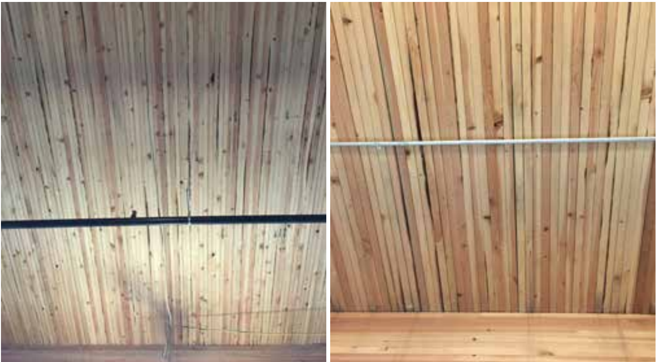
Figure A.1: Significant wane and knots, inconsistent coloration. Loose vertical tolerance on placement of laminations.
