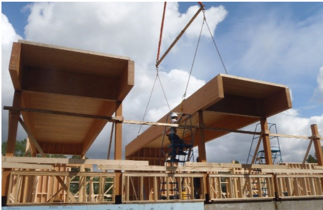
Figure 6.5: Combined NLT and support beams being installed as one. (Photo courtesy of Fast+Epp)
