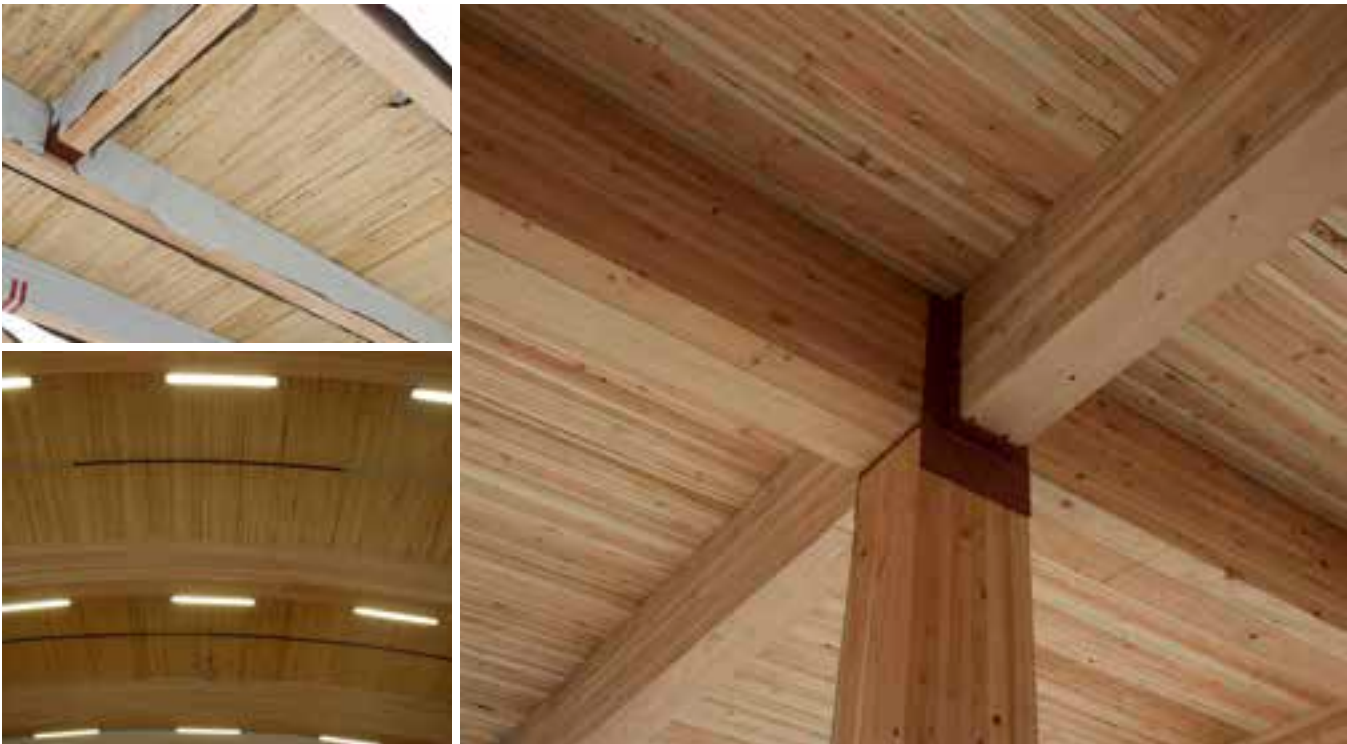
Figure A.2: Minimal wane, some knot holes, variable coloration. Tight vertical tolerance on placement of laminations.
