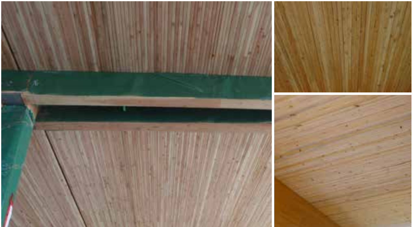
Figure A.3: No wane, minimal knot holes, variable coloration. Tight vertical tolerance on placement of laminations.
