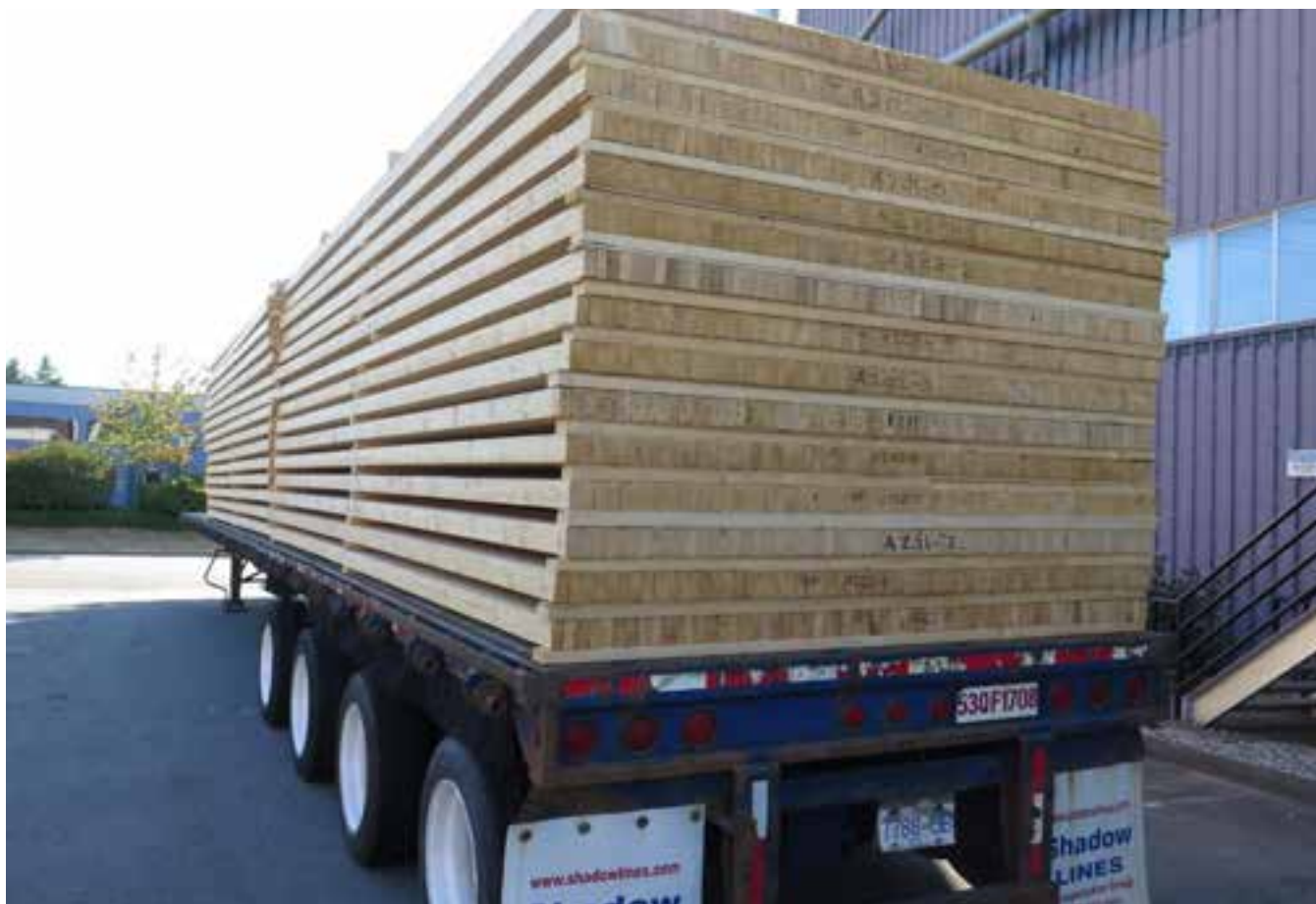
Figure 7.1: Shipping with dunnage and stickers. (Photo courtesy of StructureCraft Builders Inc.)
