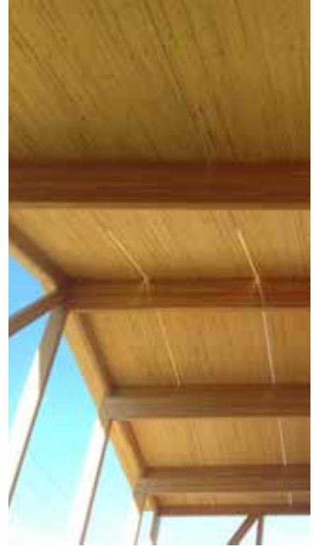
Figure 7.5: NLT install of prefabricated pre-sheathed panels. (Photo courtesy of StructureCraft Builders Inc.)
