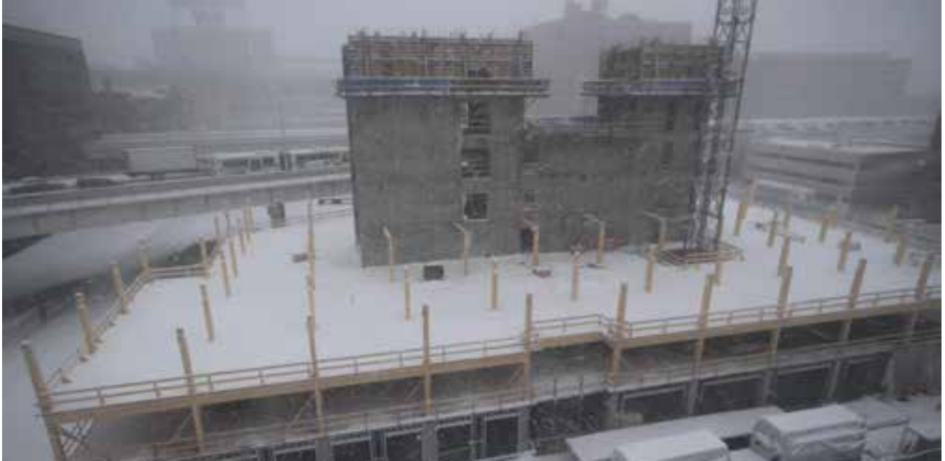
Figure 7.6: Horizontal NLT floor panel subjected to snow during the winter months in Climate Zone 6. Snow melt was later cleared from the NLT TMMS to minimize moisture exposure. (Photo courtesy of StructureCraft Builders Inc.)
