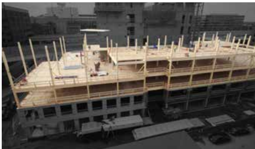
Figure 7.3: NLT panel installation sequencing model for T3 office building, Minneapolis, MN. (Image courtesy of StructureCraft Builder Inc.)
