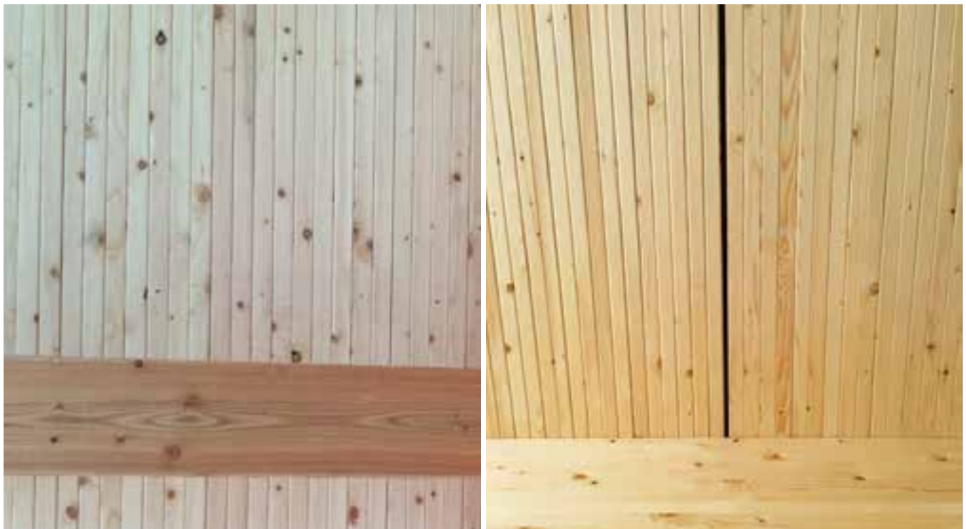
Figure A.4: No wane, no knot holes, consistent coloration. Tight vertical tolerance on placement of laminations.
